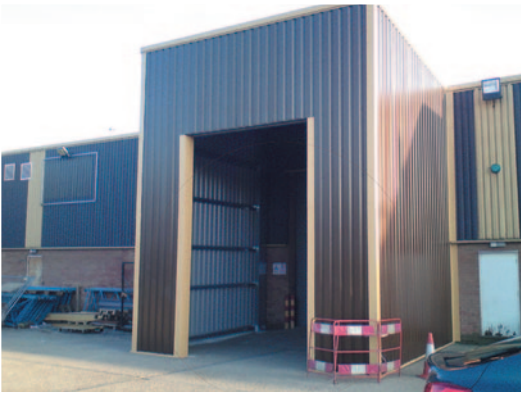
LOADING DOCK CANOPY keeping heat in and dust out of the premises
